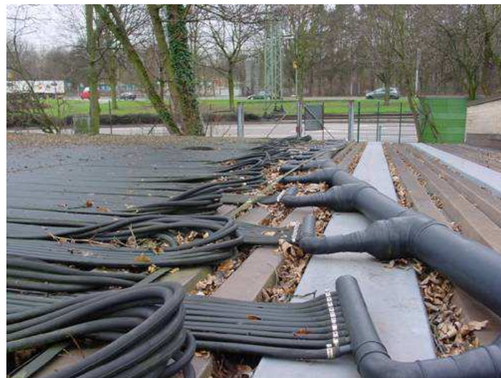
Fig. 17: Additional roof loads
