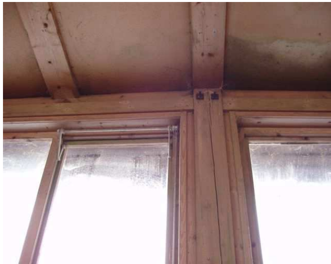
Fig. 5: Detail of connection ceiling to window frame
