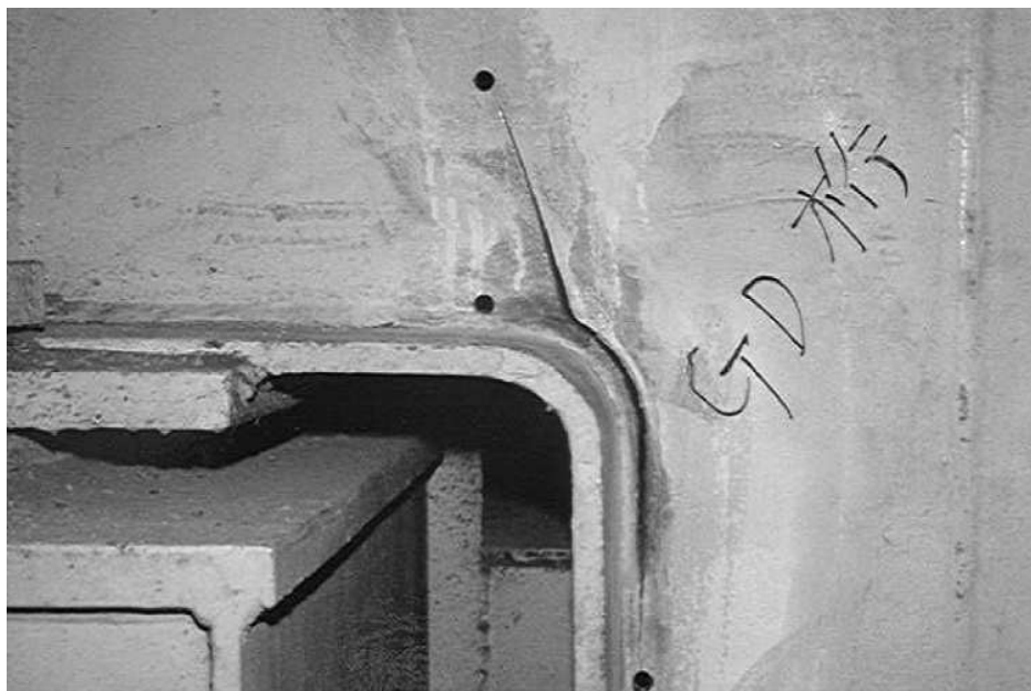
Figure 2. Fatigue Cracks in 90-Degree Rounded Detail in Japan
