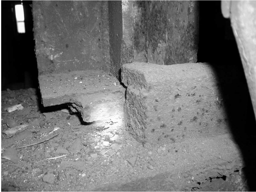
Figure 8. Corrosion of Beam Seat
