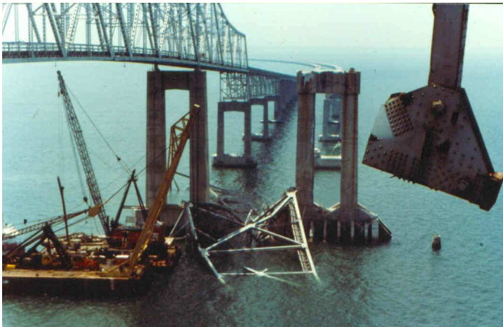
Fig. 1. View of Skyway Collapse (Courtesy of Donald F. Sorgenfrei)
