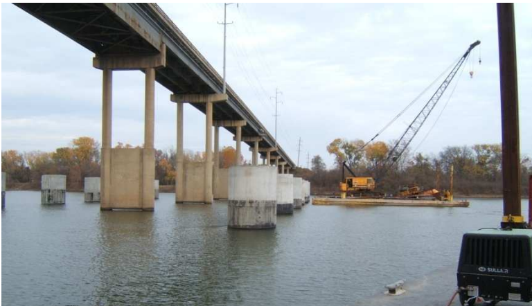
Fig. 5. Vessel Collision Retrofit (Courtesy of Jensen Construction Company)
