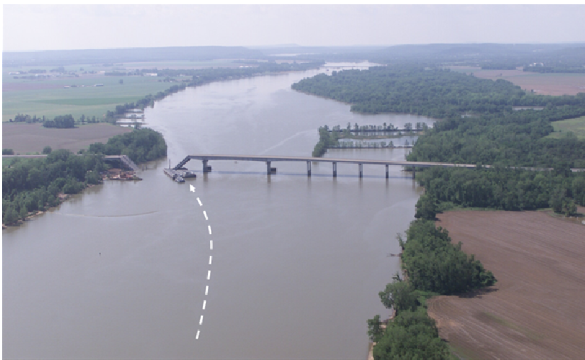
Fig. 2. Apparent Path of Aberrant Barge Tow at Webber Falls (Source: Oklahoma DOT)
