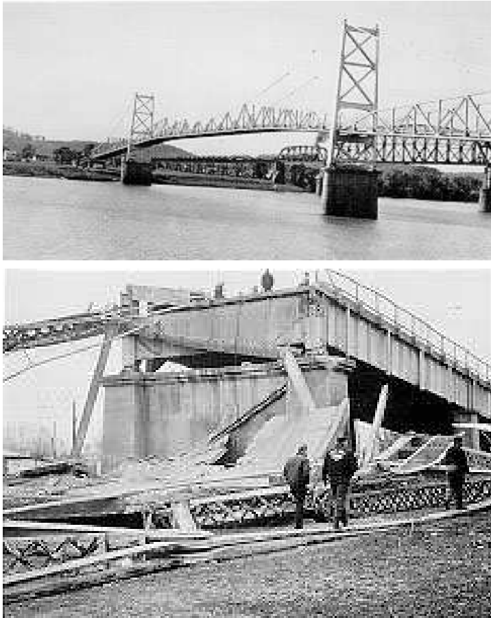
Fig. 6. Views of Silver Bridge Before and After Collapse (Courtesy of FHWA)
