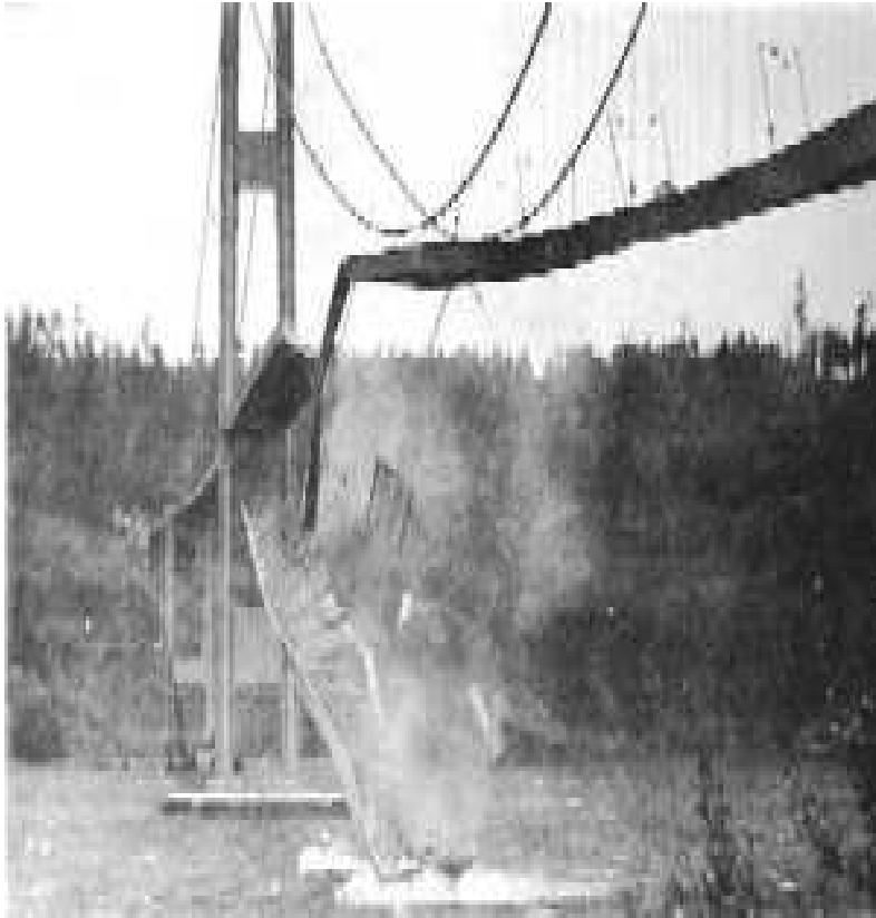
Fig. 13. Collapse of First Tacoma Narrows Bridge (Source: Britannica.com)
