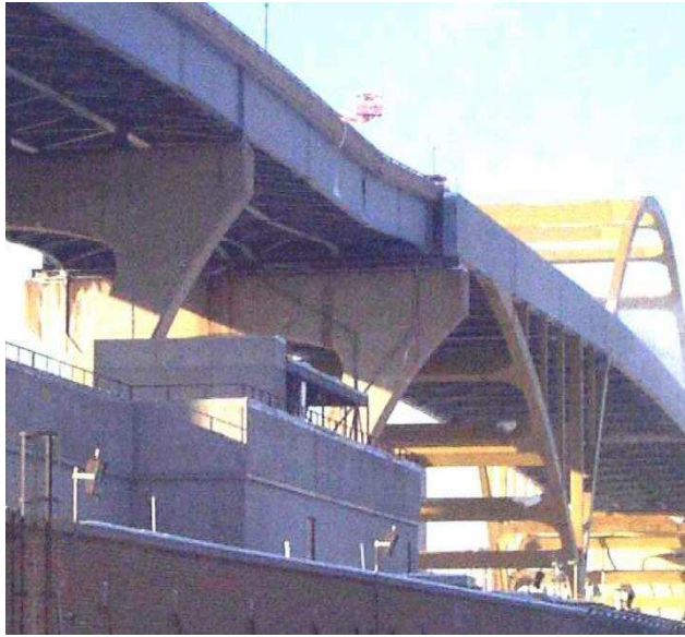
Fig. 7. General View of Hoan Bridge (Courtesy of FHWA)
