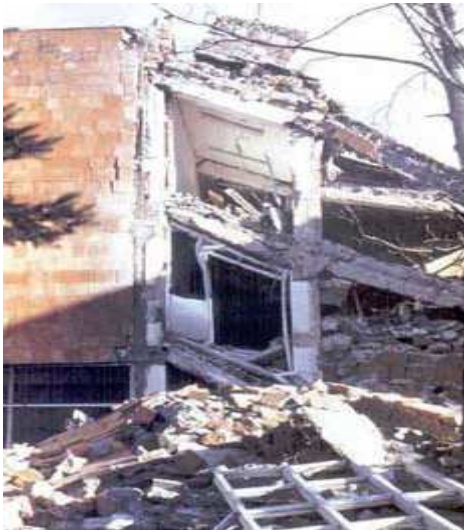
Fig. 12. Building collapse Spitak (Armenia) earthquake 1988 (WHE Report 66, Uzbekistan)
