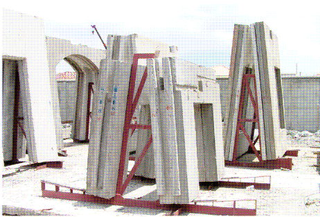
Fig. 2. Proper Storage of precast panels
