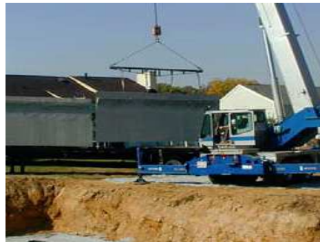
Fig. 3. Erection of precast Panels-vertically
