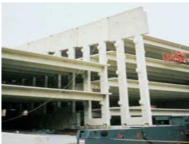
Fig. 8. A Parking Garage, Staunton, VA
