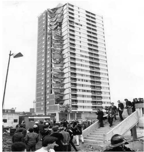
Fig. 13. Ronan Point Tower (16 th May 1968) East London (Courtesy Google web)
