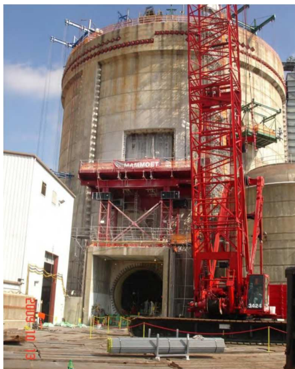
Figure 2. Original access hatch with the temporary Steam Generator Replacement opening
