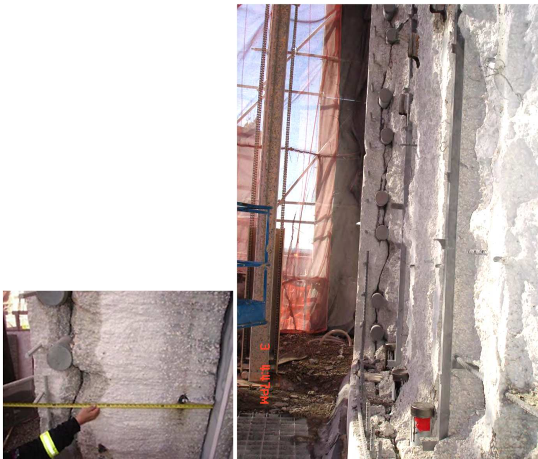
Figure 3. Delamination of concrete along the line of the prestress-tendons.
