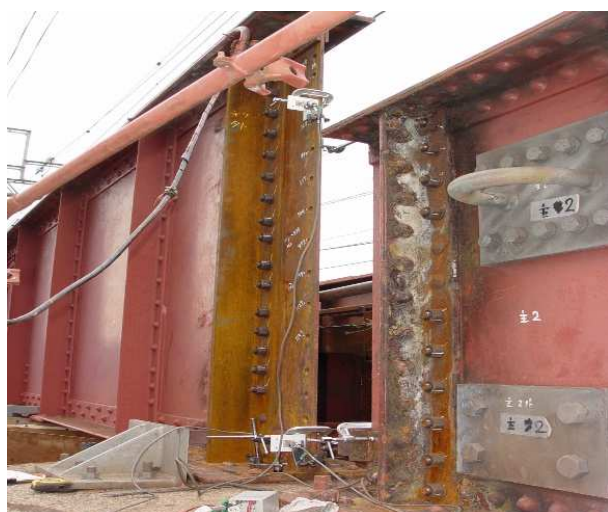
Figure 9. Installed sensors at girder ends
